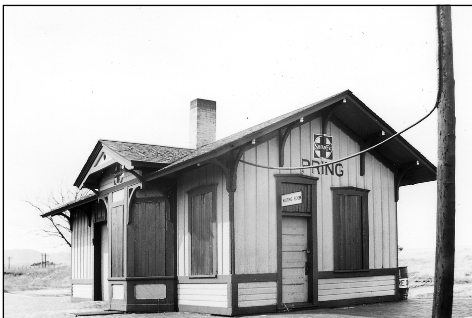
The track side and passenger end of the Santa Fe depot at Pring, Colorado, originally at MP 677.3. The 16 by 24 foot depot was built in 1888 and moved to Palmer Lake in 1938. – Three Santa Fe Railway photos, Russell Crump collection, http://www.atsfry.com
